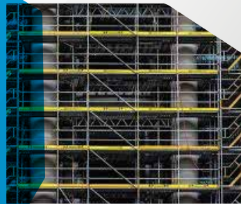
Struts, scaffolding, and trusses
